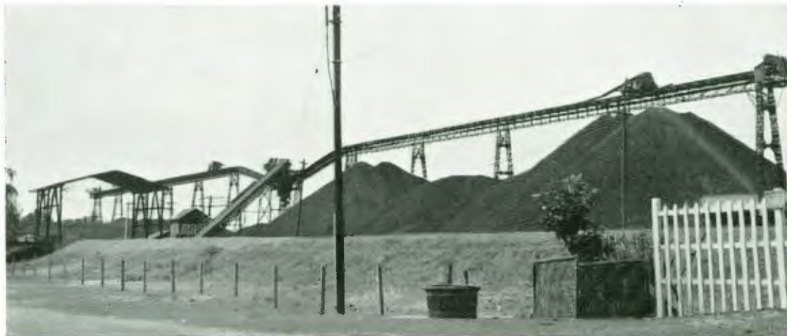
Jubakar stock pile and conveyor belt system.
